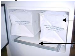
HICAP Filter Bags (AG149) located behind front access door (one for each Clearview workstation) Or one for JUNIOR unit.
